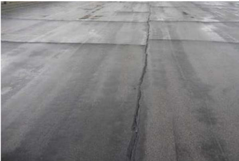
Linear Cracks
